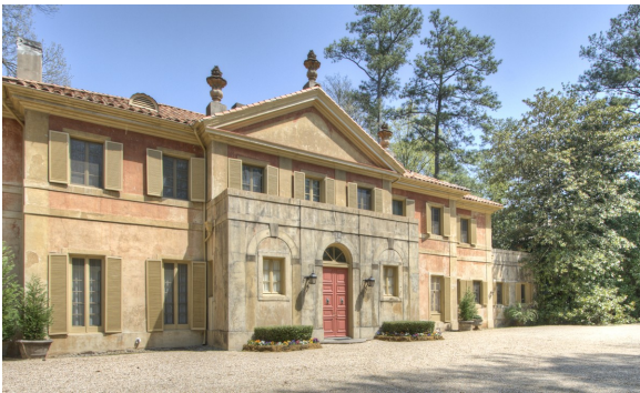
3418 Pinestream Road, NW Atlanta, GA 30327 Built in 1923 "The Pink Castle" (West Paces Ferry to Pinestream) Agent: Glennis Beacham
